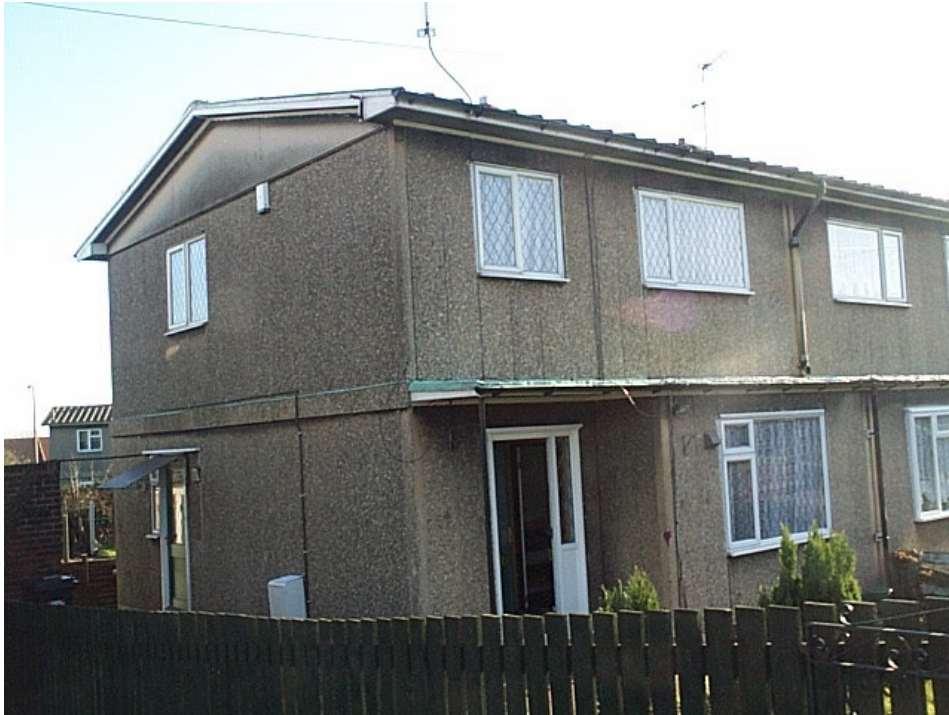
Photograph 1 – Typical Front Elevation of Tarran Newland House
